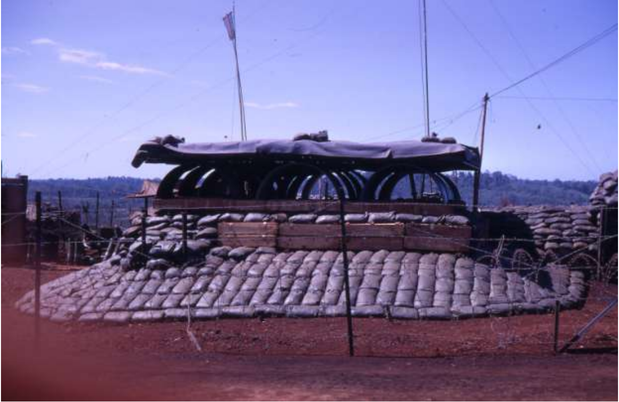
Above: FDC at Judy with standoff to explode incoming mortar rounds. Neat sandbags were done after 1 st ARVN Airborne Division took over Judy
